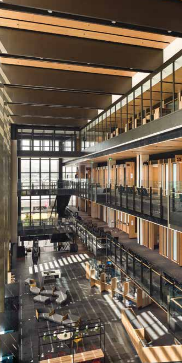
Justice and Emergency Services Precinct, Christchurch
